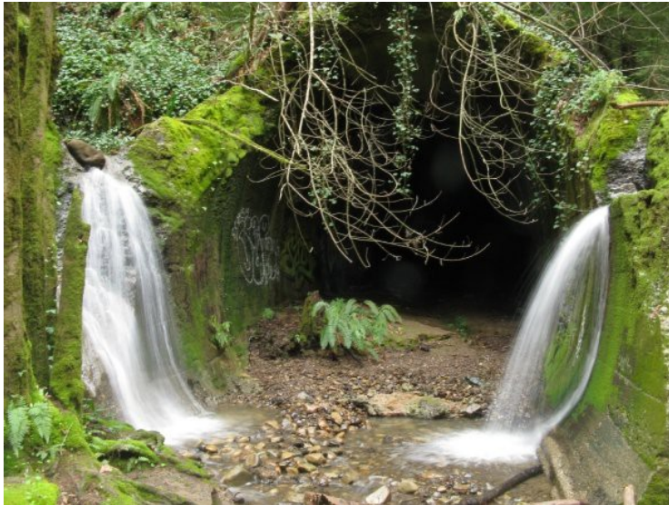
North entrance of the Wright's tunnel
