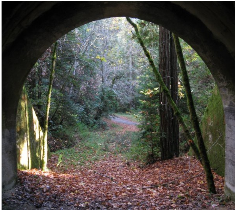
View from inside the tunnel
