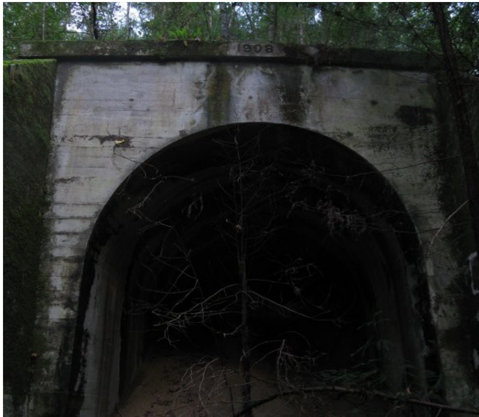
Seldom seen west end of the Mountain Charlie tunnel
