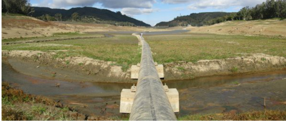
Exposed pipeline in the bottom of the empty reservoir
