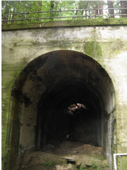
North entrance to the Laurel tunnel
