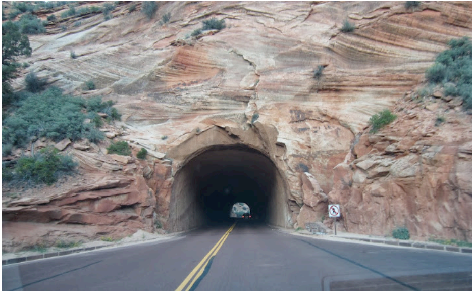
Tunnel in Zion National park
